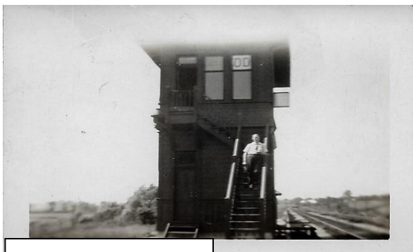
Curtis McConoughey at switch tower
